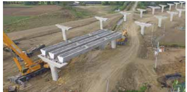
Road construction linking Ratchaphruek and Kanchanaphisek roads (north-south)
