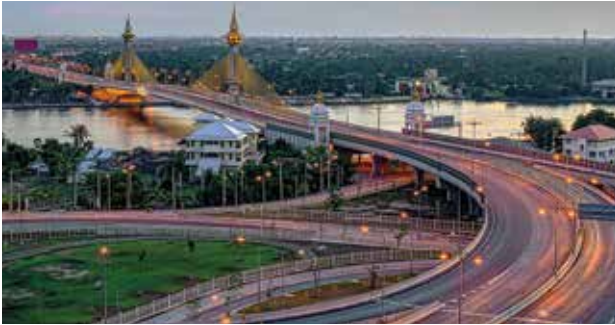
Maha Chesadabodindranusorn Bridge
