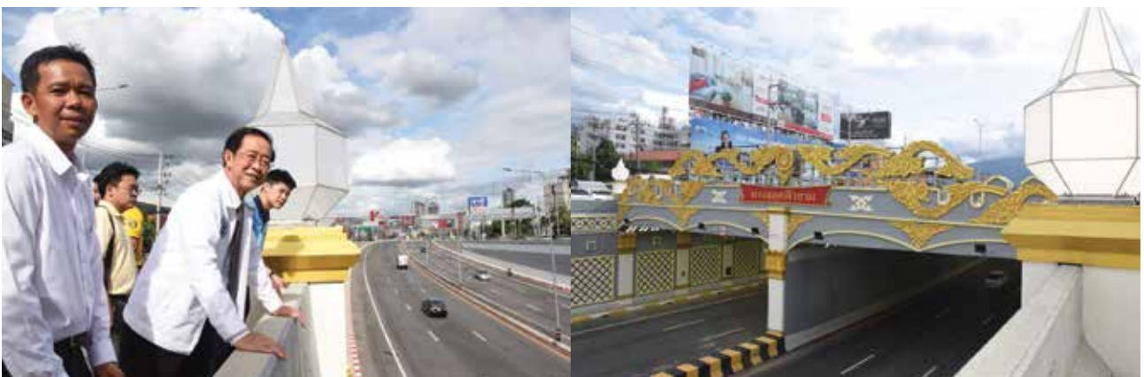
Mr. Arkhom Termpittayapaisith, Minister of Transport, inspected operational readiness of the Project of Traffic Improvement and Accident Mitigation of Fah Ham Underpass Traffic Control and Facilitation Building on 8 June 2018.
