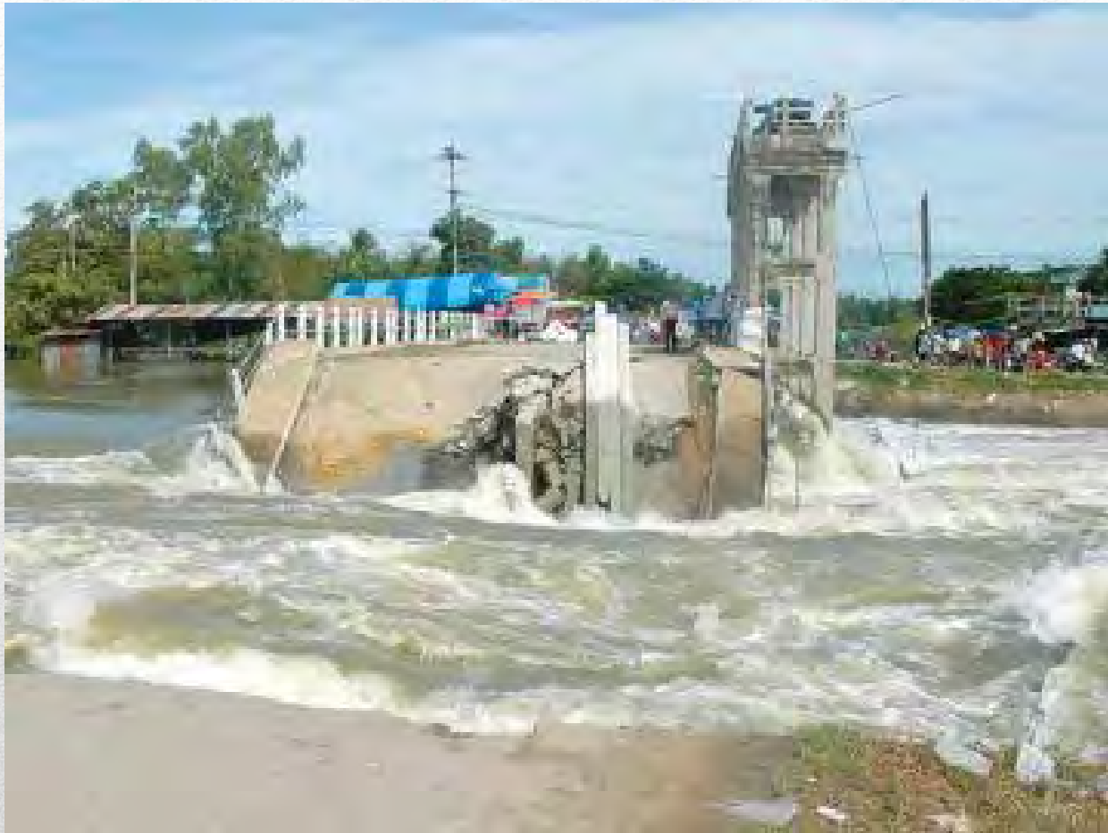
Broken sluice
